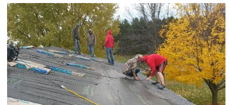
Students working together to shingle a roof.
