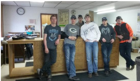
Dylan Sexton, Reid Winkler, Dylan Krueger, Trevor Kohls, Tristen Francois, and Jon Heoft after installing the new counter at Gillett Milling.
